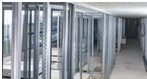
Drywall tracks to concrete and steel
