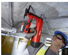
Threaded rod attachments to concrete
